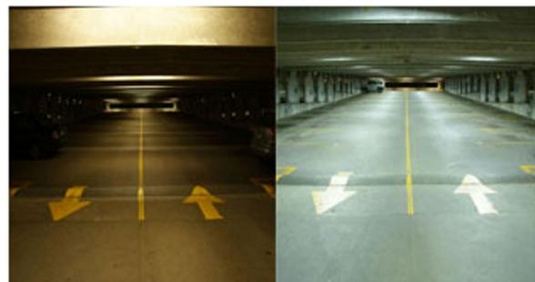
Parking station fluorescent lights (left) replaced by LEDs — increased visibility, decreased energy and maintenance costs<sup>iv</sup>.
